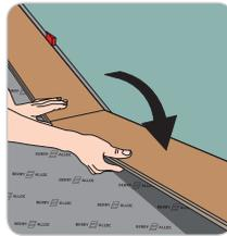
For the most natural floor pattern, make sure to mix the designs of the planks across the floor. The end joints should be staggered min. 1/3 of a plank when installing the floorboards. The first and the last floorboard in each row should have a minimum length of 1/3 of a plank.
